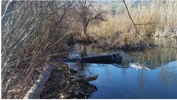
Figure 1. a) Upstream and b) downstream view of the pond leveler installed in the McDougall Wetland beaver dam.
