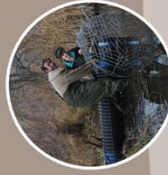
Irregular shaped fencing upstream of culverts keeps beavers from blocking them.
