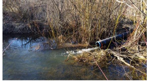
Figure 1. a) Upstream and b) downstream view of the pond leveler installed in the McDougall Wetland beaver dam.
