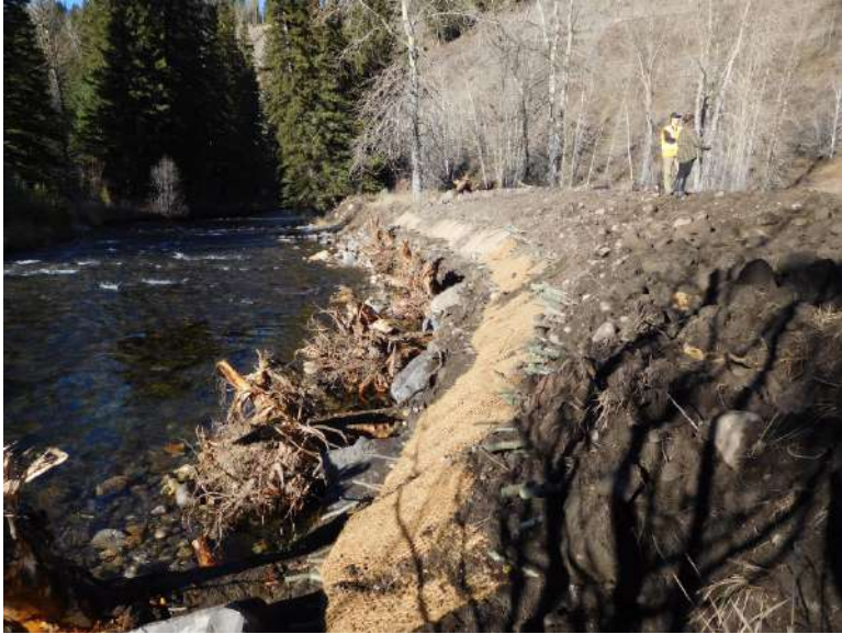
Figure 23: Completed bank stabilization and slope re-contouring
