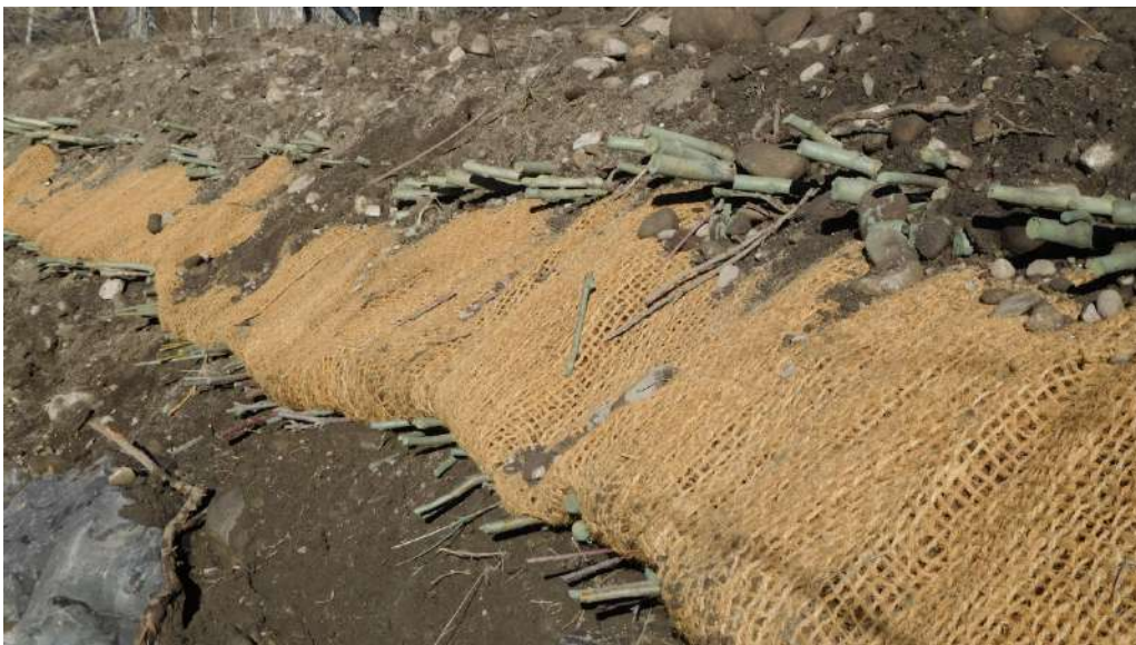
Figure 22: Coir matting securing soil between brush layers
