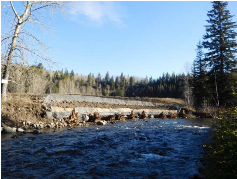
Figure 29: Completed streambank stabilization project a restoring 30 m stretch of eroded bank
