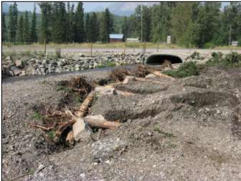
Figure 2. Example of rootwad and footer log construction before backfilling.
