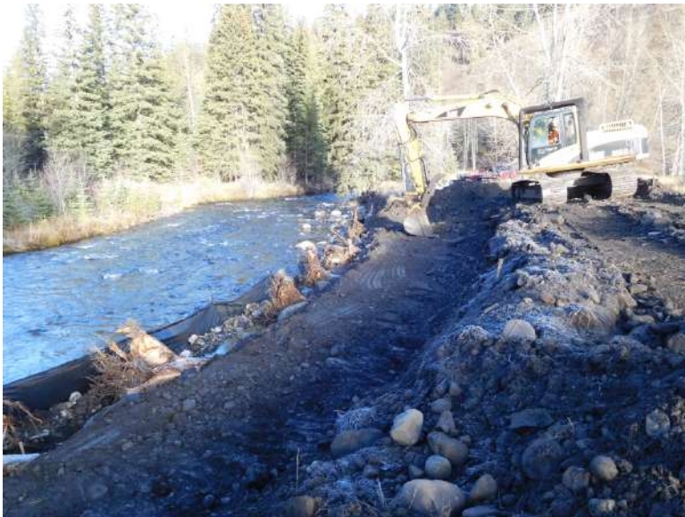
Figure 20: Excavated bench for first brush layer
