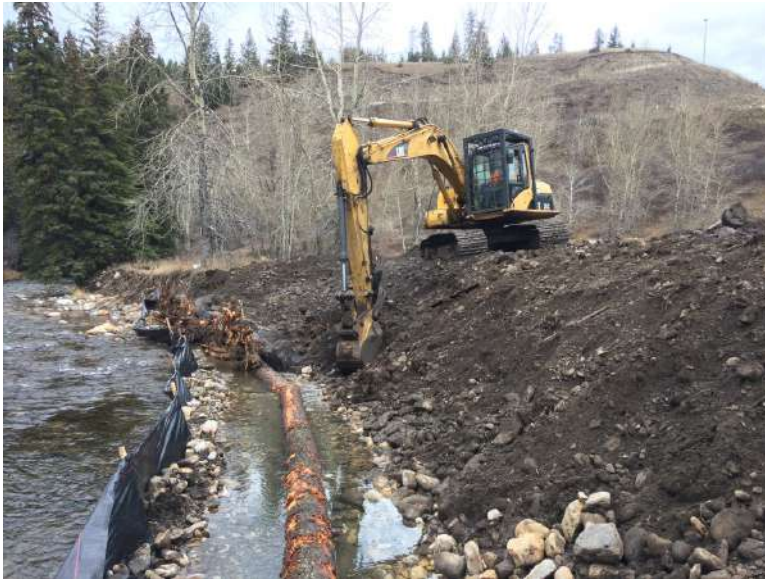
Figure 10: Excavator placing footer logs in trench
