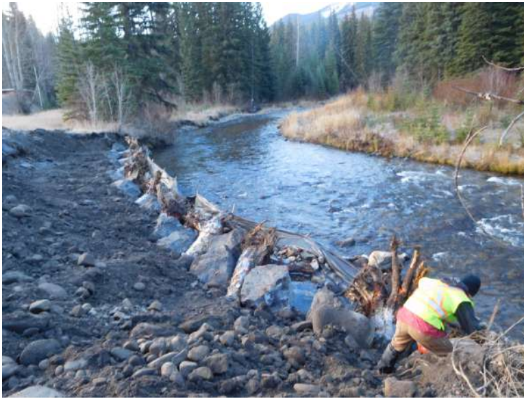
Figure 12: Rootwads secured with boulders above footer logs
