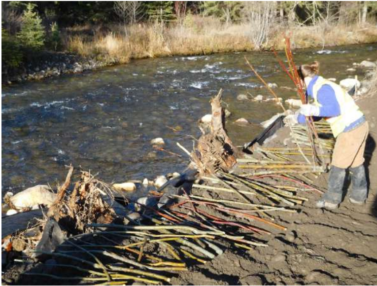
Figure 21: Placing cuttings on the bench
