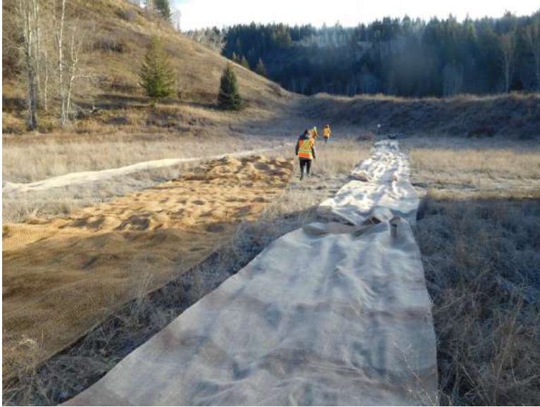
Figure 19: Cutting the coir matting to length
