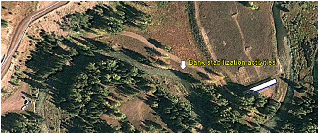
Figure 3: Specific location map showing aerial view of the project site
