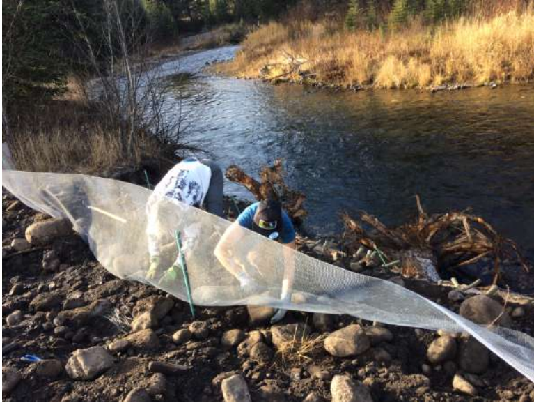
Figure 25: Rodent fence installation
