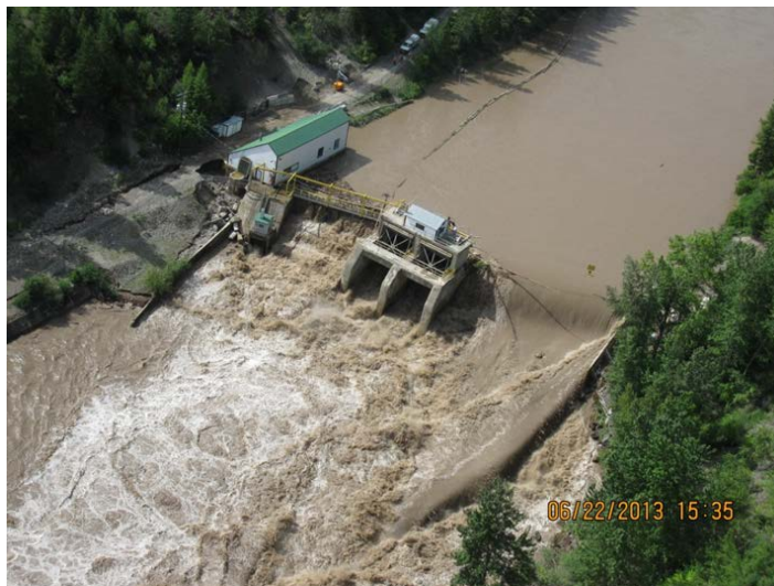
Figure 17. Elk Dam, June 2013. Credit: Dwain Boyer
