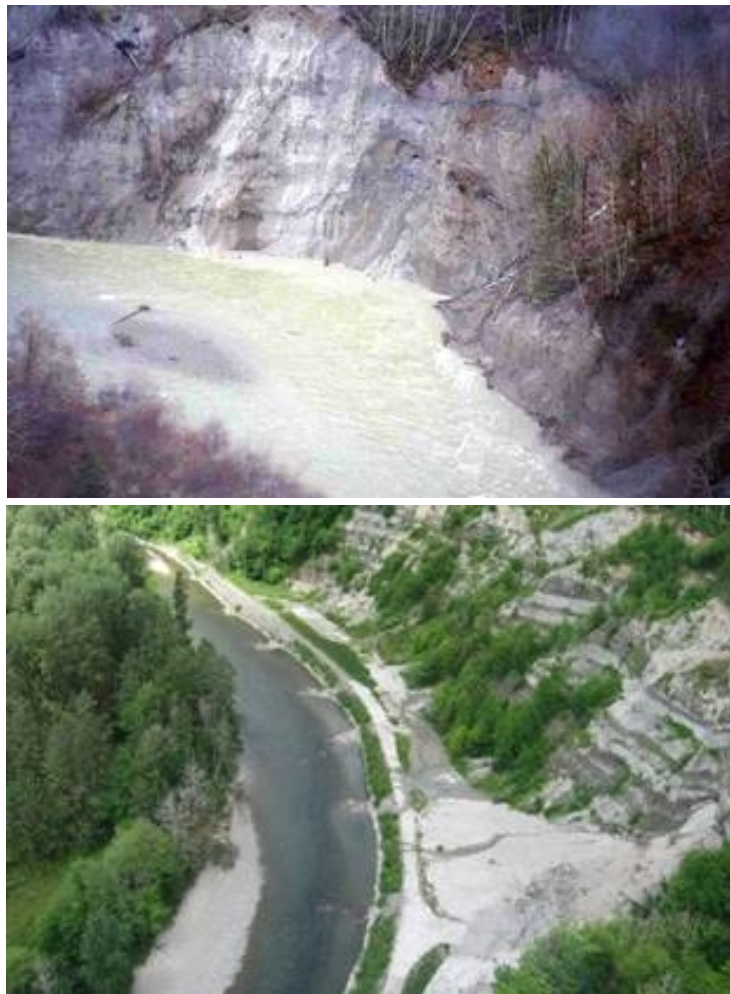
Figure 40. Stoltz bluff before and after bank stabilization project. Credit: Kerr Wood Leidel.
