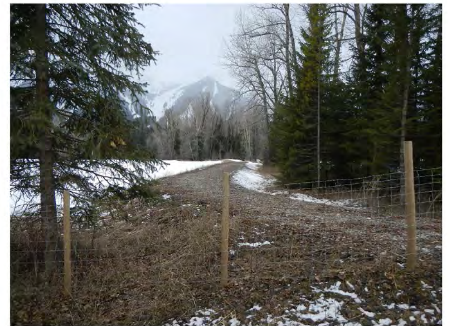
PHOTO 2: DOWNSTREAM VIEW OF EXISTING BERM CONSTRUCTED POST-2013.
