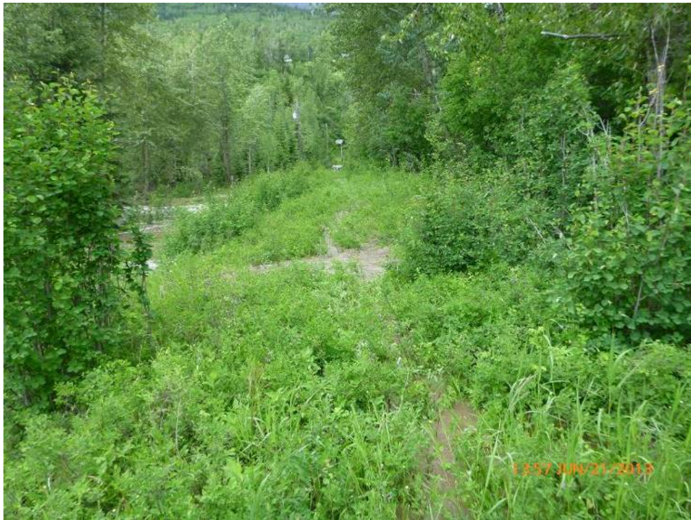
Figure 11. Water overtopping dike in June 2013 (source: RDEK).
