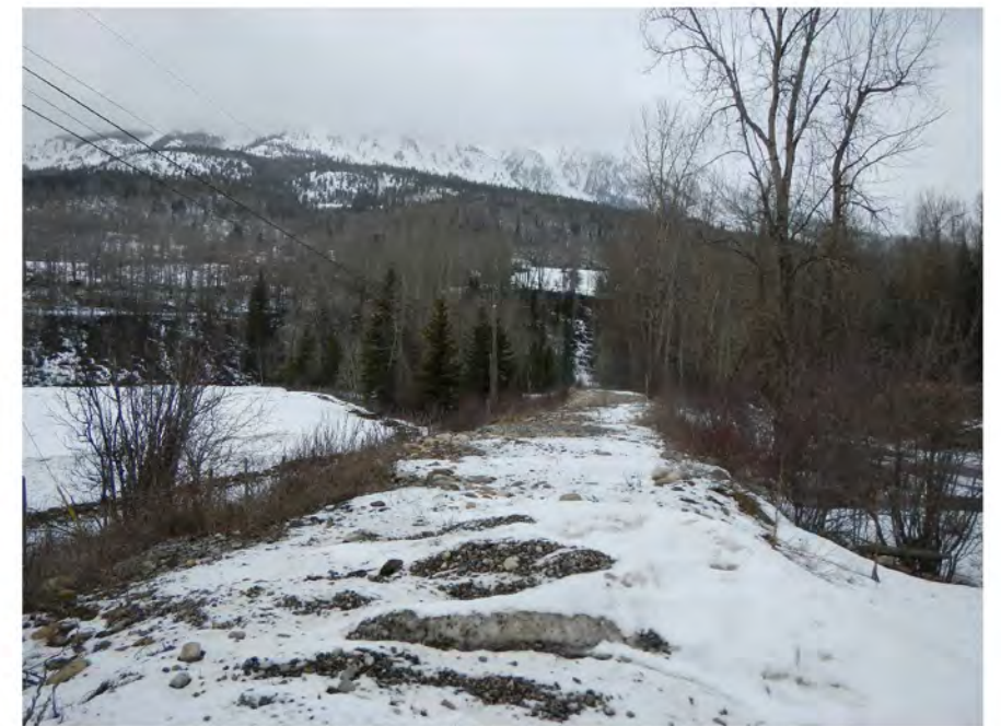
PHOTO 1: VIEW OF EXISTING DIKE FROM HIGHWAY 3.
