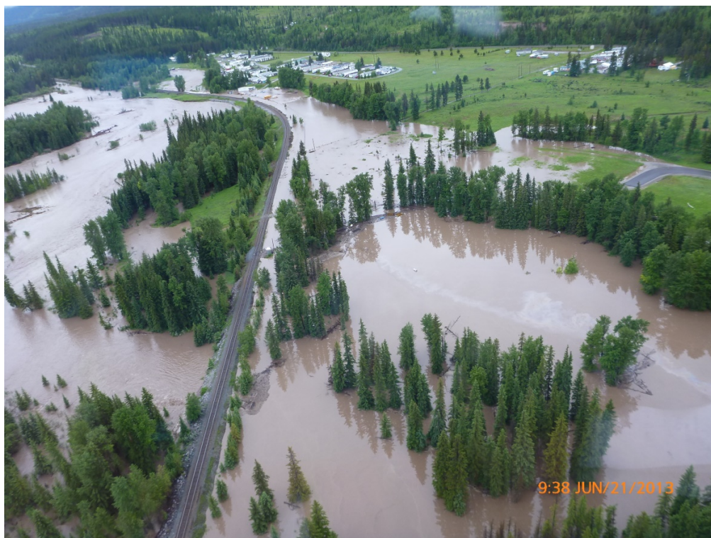
Figure 2. Whispering Winds Trailer Park during June 2013 flooding (Source: RDEK).
