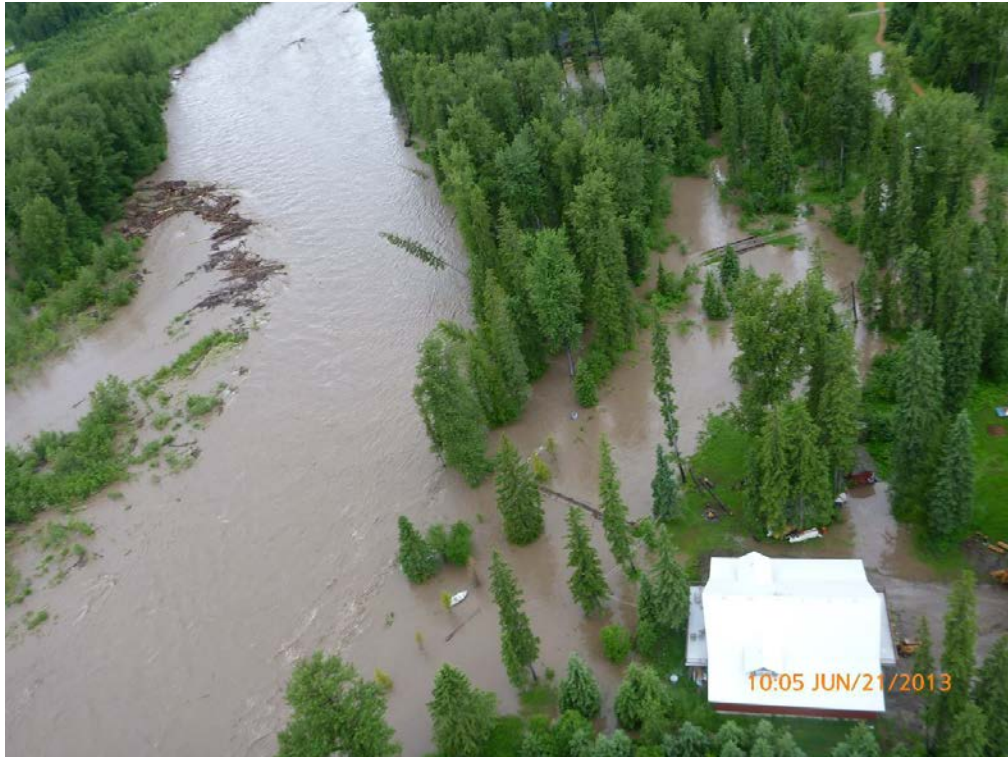
Figure 24. Properties adjacent the Elk River along Thompson Road during the June 2013 flood.
