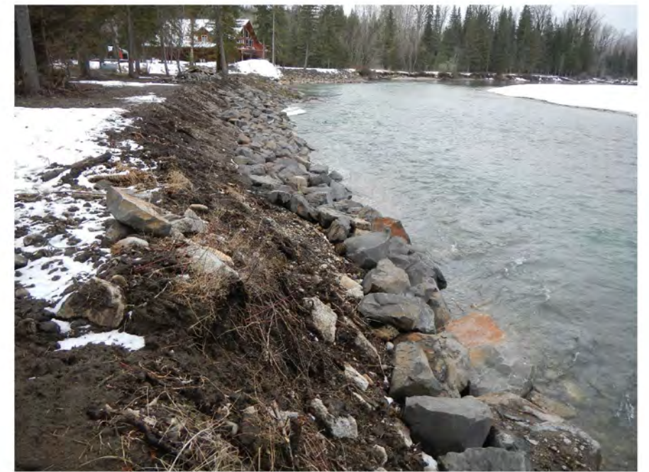
PHOTO 1: DOWNSTREAM VIEW OF EXISTING RIP RAP WORK.
